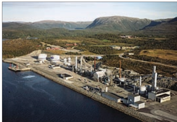
An overall view to a liquefier in Norwegian Tjeldbergodden.
