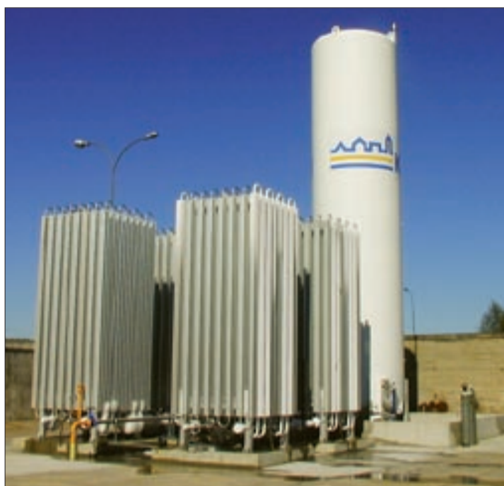
Installation of an LNG vaporization unit for KRI Poland.
